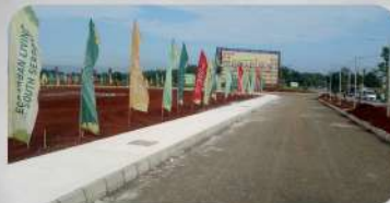
Progress Group Bogor - Jawa Barat - House Development
